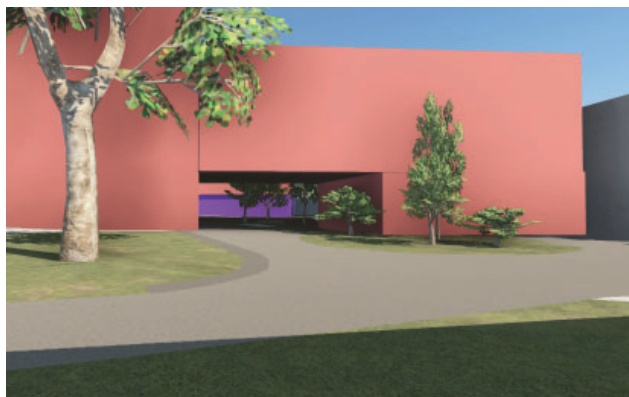
5. View from the front of Grade II listed Beam Engine Houses
