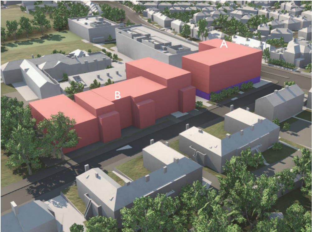
Aerial view from the south-east
