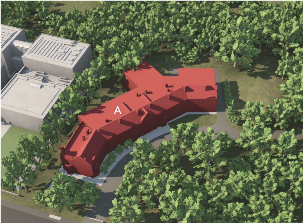
Aerial view from the south-east
