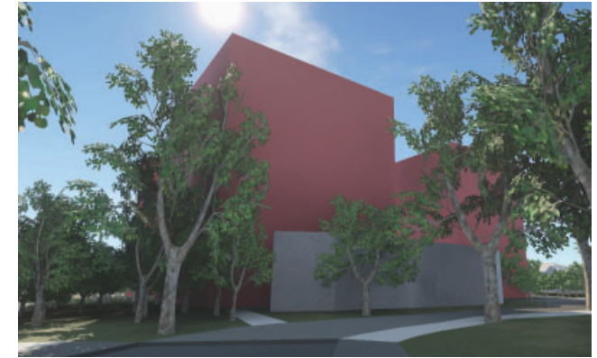
2. View from south east entrance
