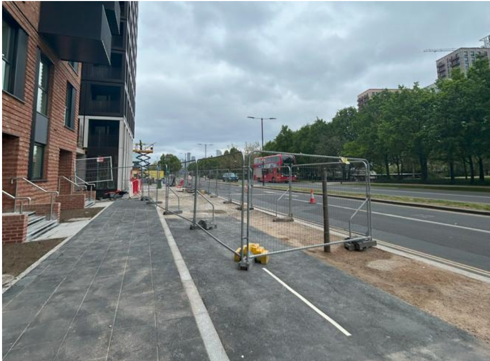
Figure 61: View along West Parkside in North Greenwich towards the O2 Arena
