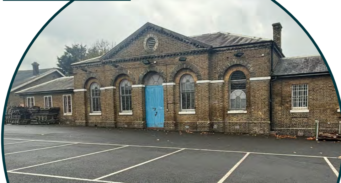
Figure 26: Grade II listed Gun Park Block, Upper Gun Park
