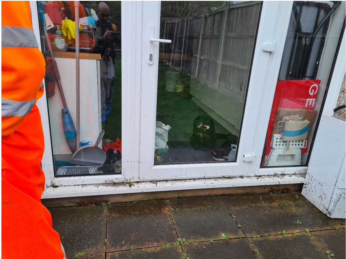
Photograph 2 Rear of property on Woodbrook Road (07.11.2022)
