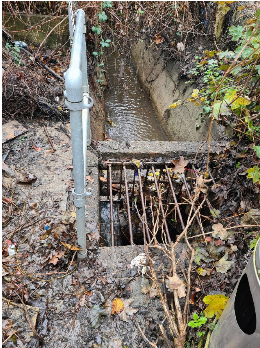
Photograph 6 Alternative view of screen (29.11.2022)
