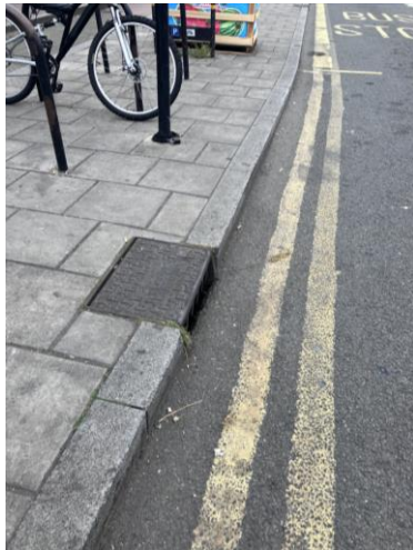
Photograph 16: Road gullies with wide openings which are known to become blocked at location of flooding
