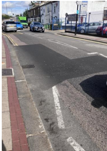
Photograph 20: location to remove swan neck outlet and add additional road gully.
