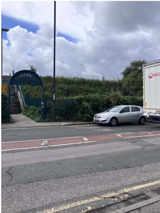
Photograph 10: Low point on Nathan Way adjacent to footpath over the Ridgeway
