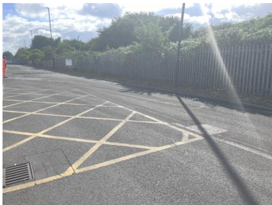
Photograph 11: Entrance to Greenwich Reuse and Recycling Centre
