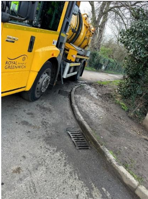
Photograph 6: Three gullies at the junction between King John's Walk and the public footpath
