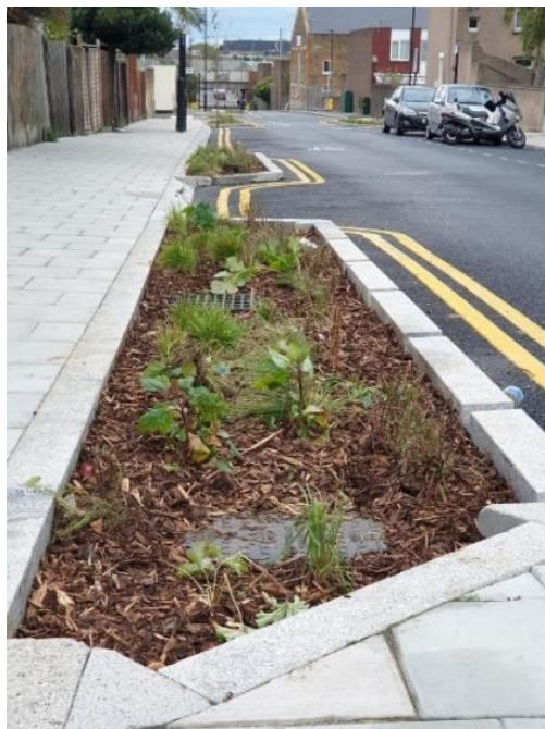
Photograph 13: Rain gardens on White Hart Road
