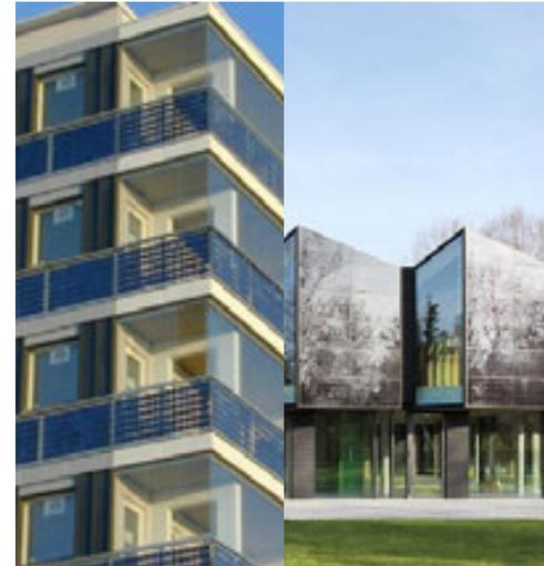
✔ Image f.73: BIPV can be successfully expressed into a range of building elements, including wall-cladding, balustrades of balconies and window glazing.
