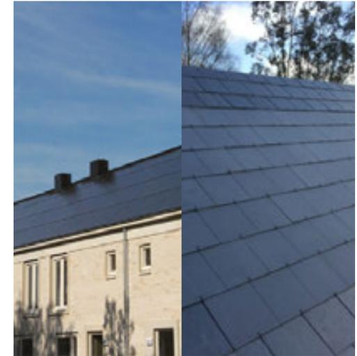
✔ Image f.74: PV panels can successfully replace other materials on the roofs and canopies. Other products suitable to historic buildings are available, including solar slates systems.
