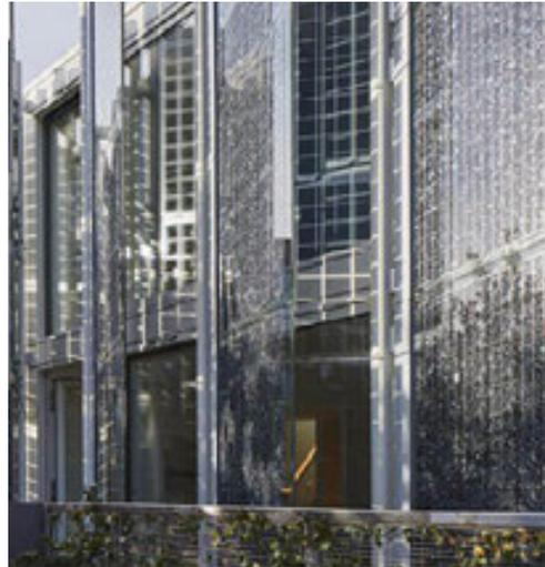
✔ Image f.72: PV double skins can address overlooking issues on constrained sites and provide expressive light/shadow effects on facade - Example: 740 Fulham Road - HCL Architects
