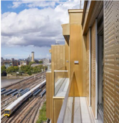
✔ Image f.67: Operable screens and shutters in front of windows are much more effective than internal shutters in avoiding the overheating of indoor space. They also facilitate customising the level of natural light to the residents' needs and reducing exterior noise.
