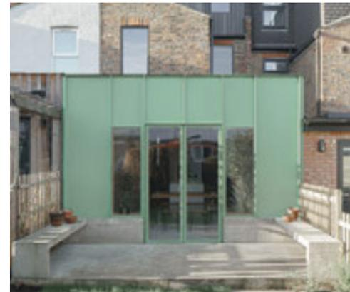
✔ This contemporary extension, uses tonal metal cladding to contrast with the original brickwork. It retains a high level of privacy through more modest glazing, while blending into the garden through a subtle concrete banding. | deDraft, Photographer: Nick Dearden
