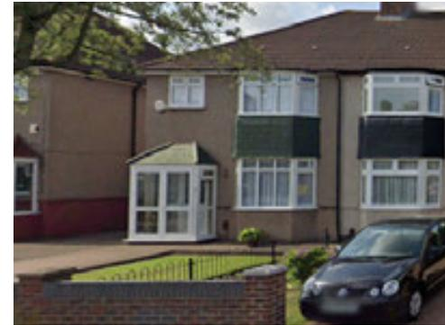
The front extension on the left hand side is kept separate from the projecting bay window. It uses similar colours and materials.
