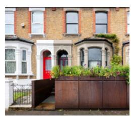
Image d.36: Cycle storage integrated into the boundary wall (image from **BikeBox Works)**
