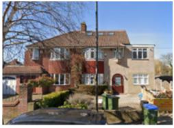
A two storey side extension impacts on neighbouring amenity. In this example there is no set back from the original front facade which results in breaking rhythm of the streetscape. The roof is flat, not following the pitch of the original roof, making the extension look out of place.
