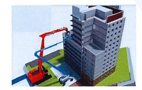
Structures will be demolished via controlled removal of sections of each building, ensuring safety and minimising disruption
