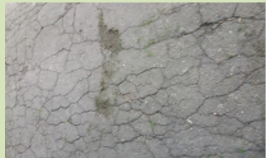
Degraded surfacing at Shrewsbury Park
