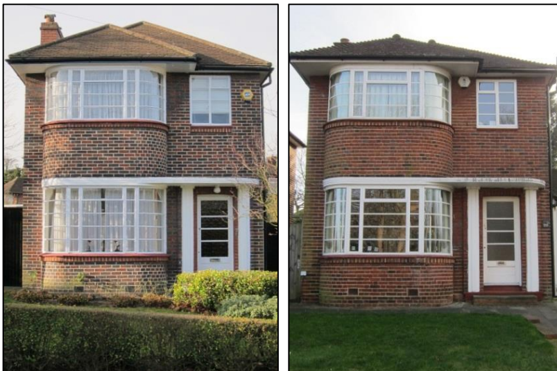
Figure 6: Type 3 Moderne style curved front bay (width type 1): original (left); and reproduction retaining original proportions (right)
