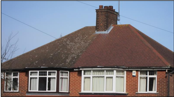
Figure 1: original (left) and replacement (right) concrete tiles (concrete will weather to match)
