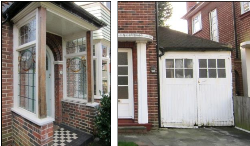
Figure 10: (left) original porch design (used on Aberdeen and Rona Deluxe houses) and (right) original garage with hipped roof and part glazed doors
