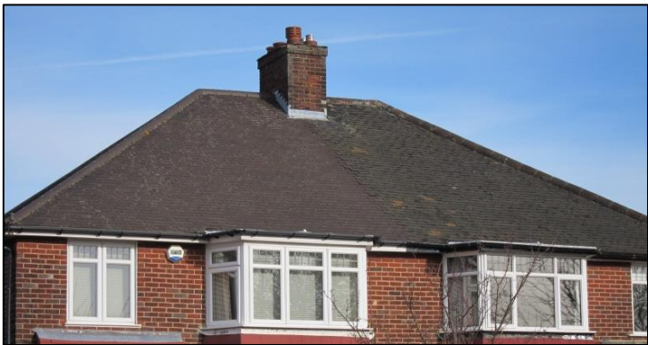
Figure 2: original (right) and replacement (left) clay tiles
