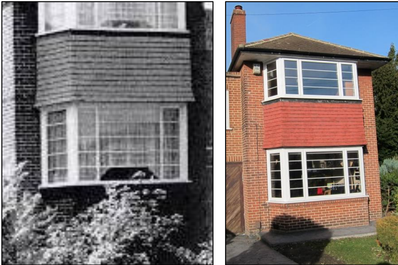
Figure 7: Type 2 Moderne style angled front bay: original (left) and reproduction (right)
