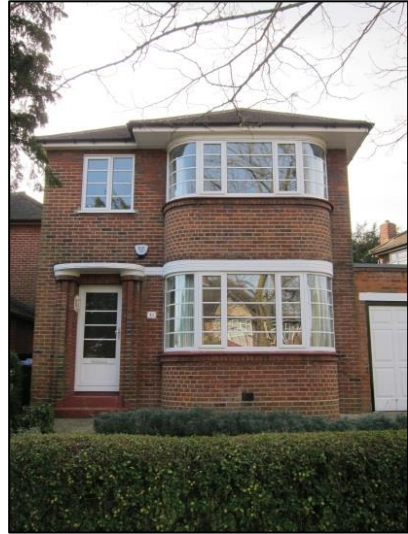
Figure 9: Type 3 Moderne style curved front bay (width type 2): original (left) and reproduction retaining original proportions (right)
