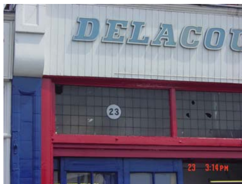
Fig 2 & Fig 3: 21- 25 Delacourt Road with close-up of shopfront showing old joinery and replacement fascia board
